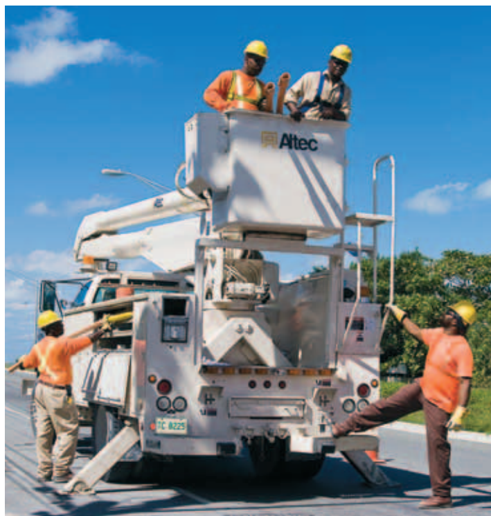
Fortis Turks and Caicos has a combined diesel-fired generating capacity of 48 MW and met a combined peak demand of 28 MW in 2007.
