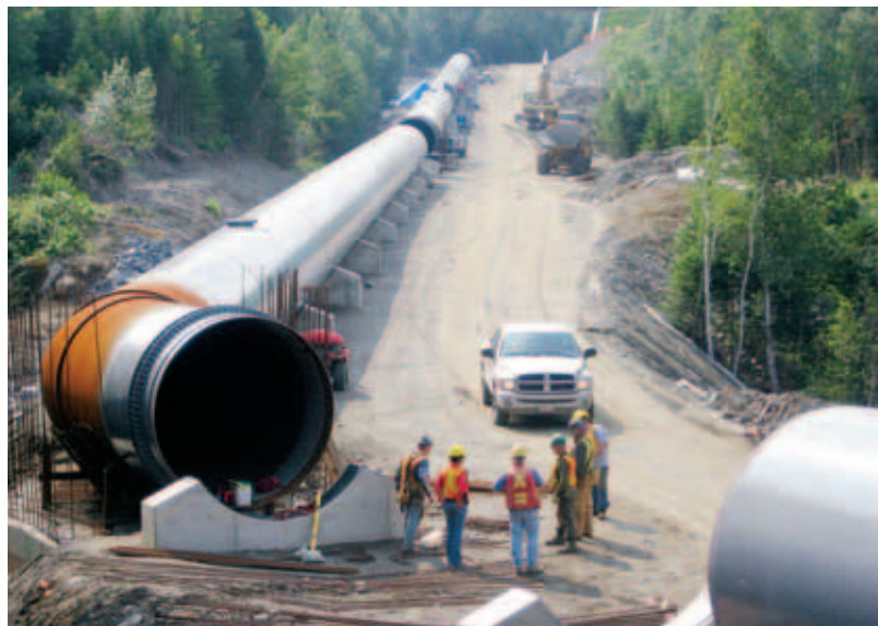
A $17 million refurbishment of the Rattling Brook hydroelectric generating facility, the largest capital project in dollar terms ever undertaken by Newfoundland Power, was completed in 2007.
